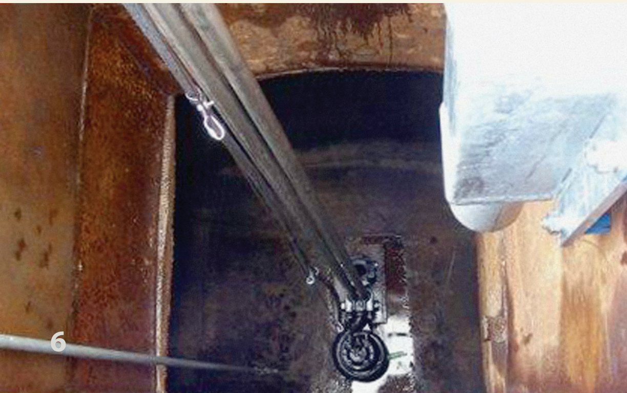
Chopper submersible pump installation with foot coupling.
