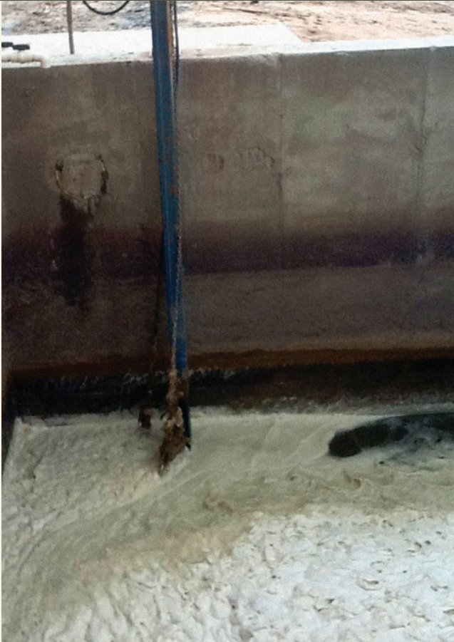
TBM mixer installed in waste water pit.
